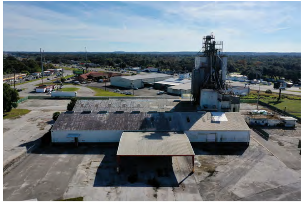
Aerial Facing S
