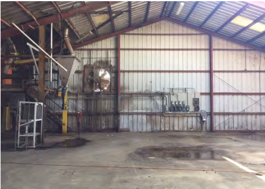
Large Mill Cooler and Screener Area
