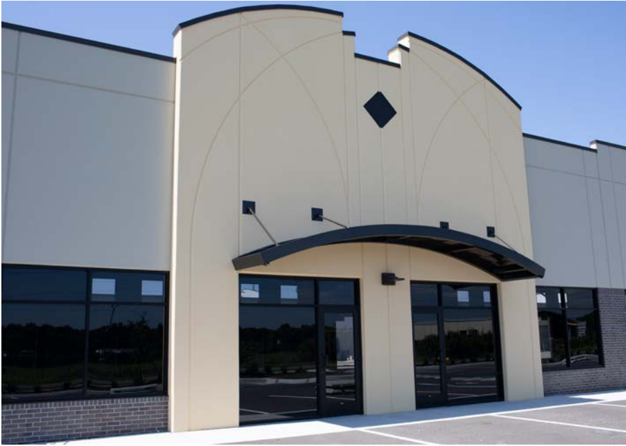
Exterior Construction Update (6-10-2020)
