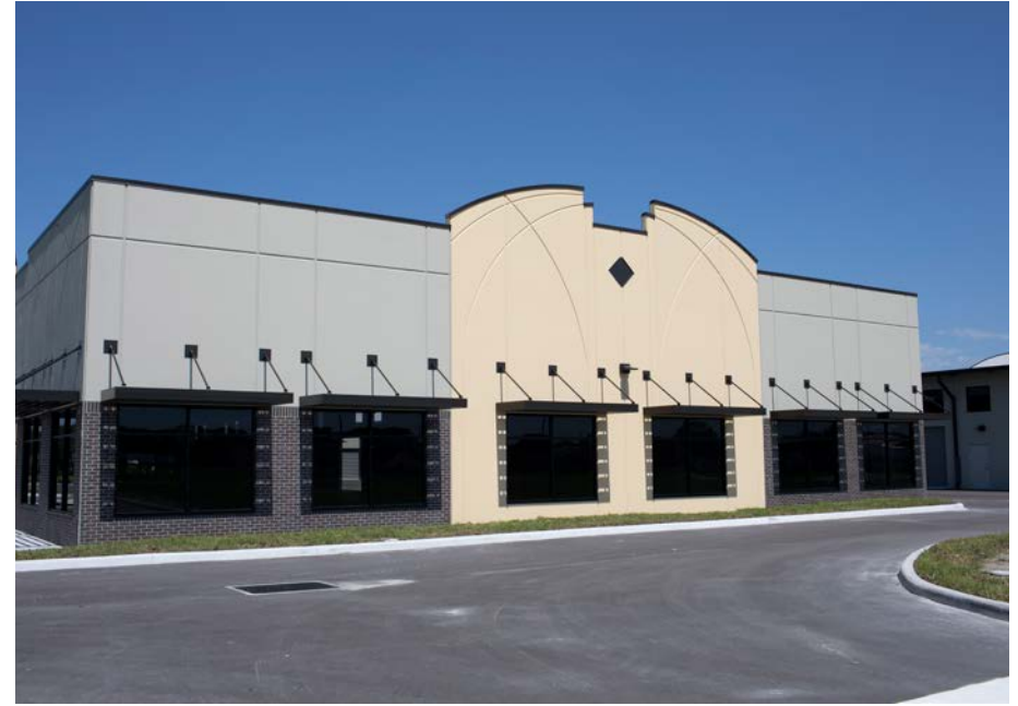
Exterior Construction Update (6-10-2020)
