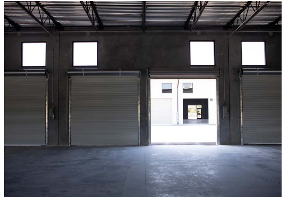
Interior Construction Update (6-10-2020)
