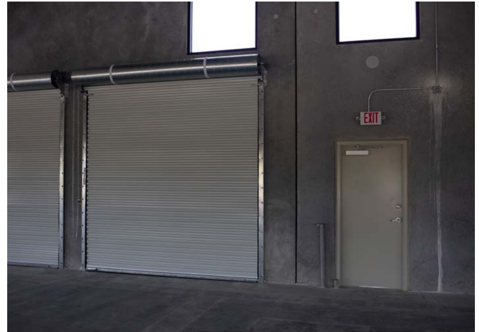
Interior Construction Update (6-10-2020)
