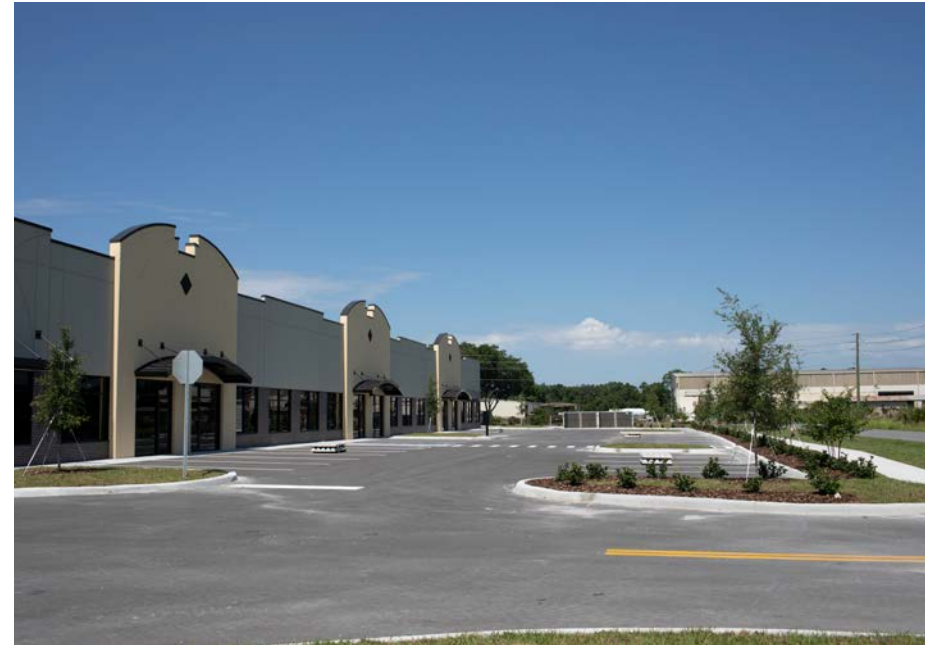
North building parking area
