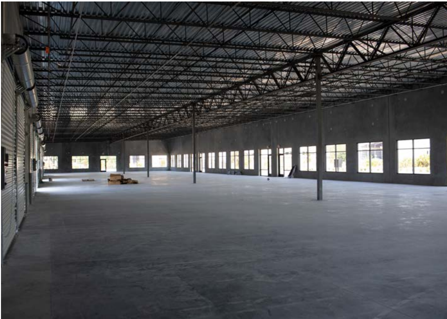
Interior Construction Update (6-10-2020)
