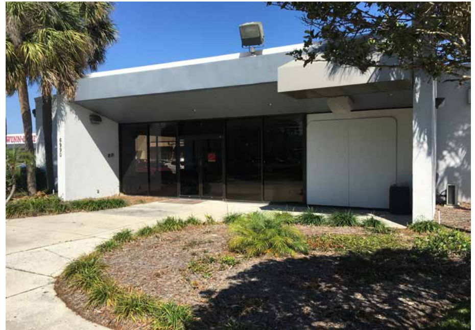
Front door entrance
