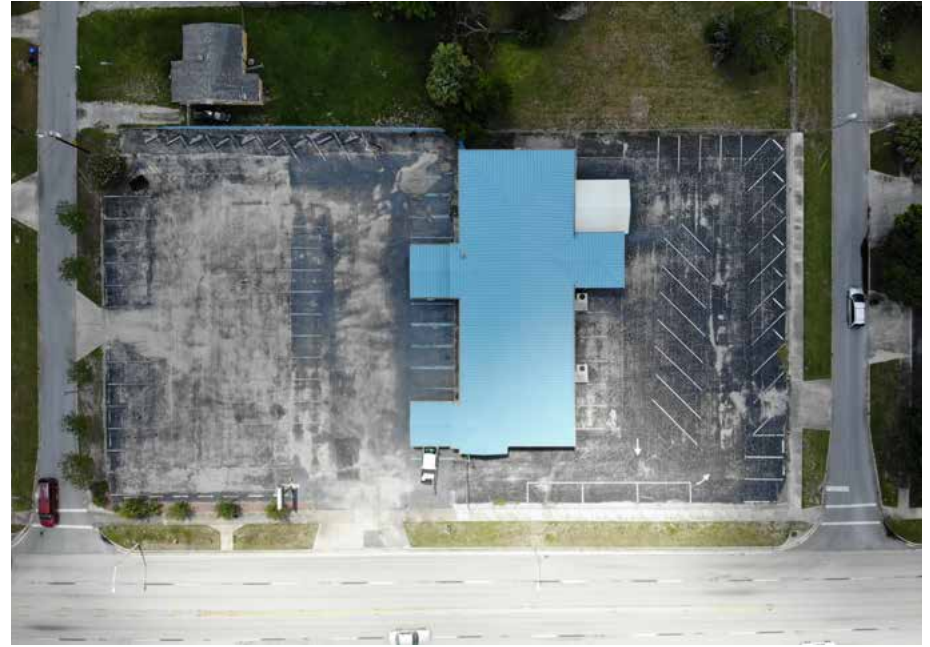
79 parking spaces around the building
