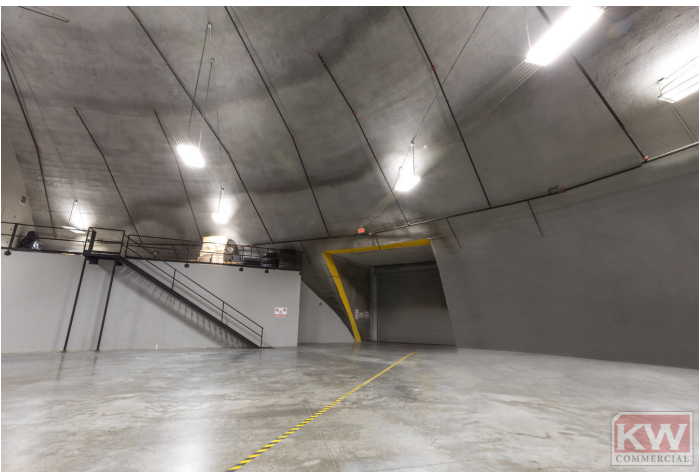
Dome B - Warehouse space
