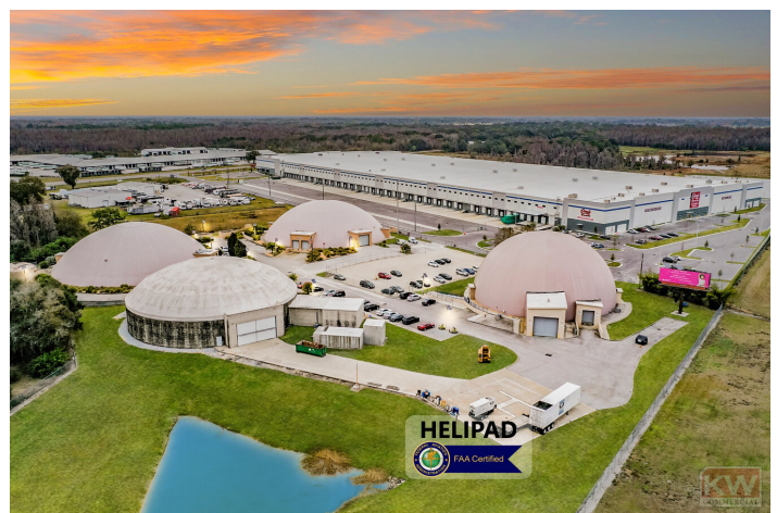
Aerial View - Helipad on site
