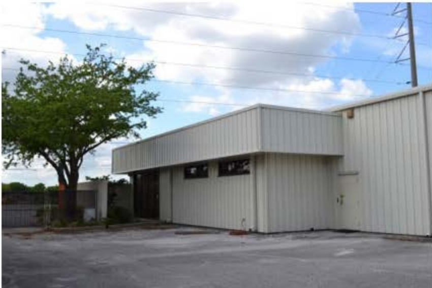
South Side of Office
