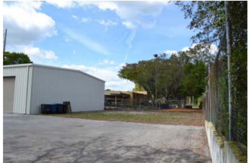
Back of Warehouse
