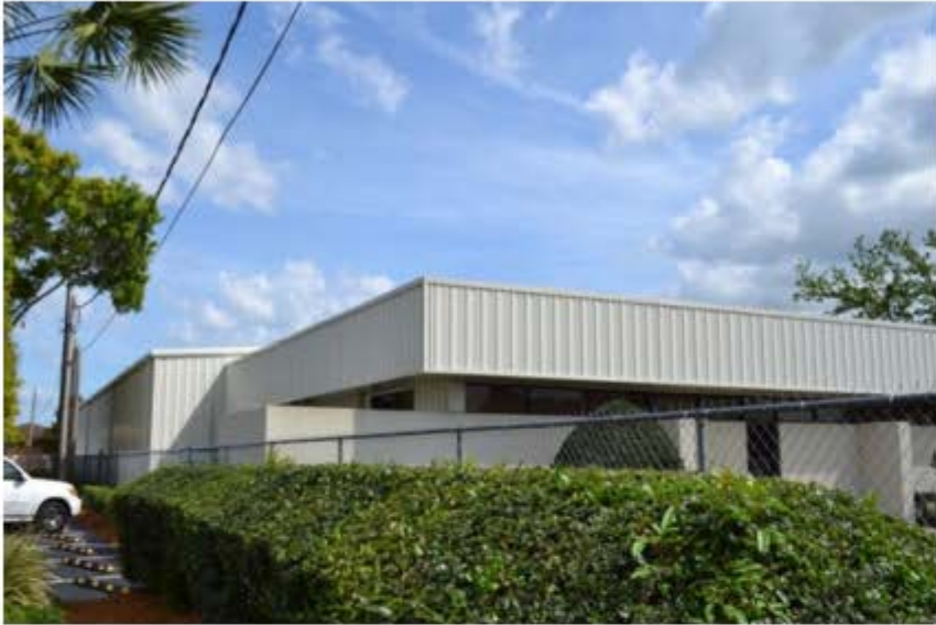
North Side of Office
