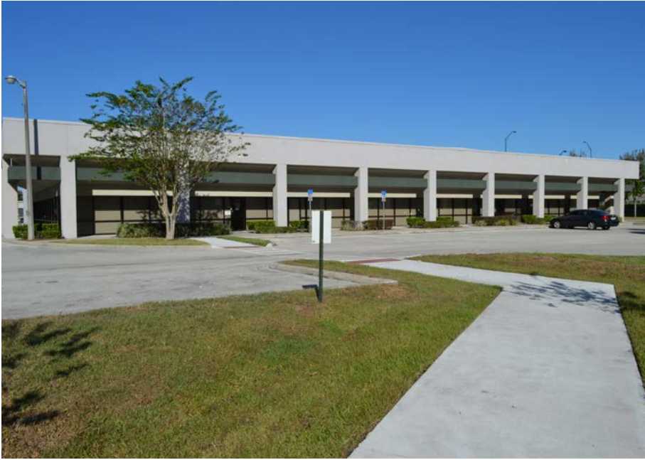
Ground-view of Building 1
